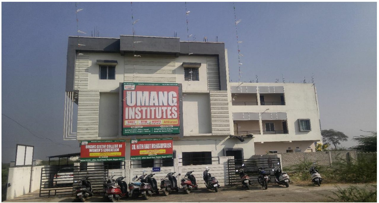
College Building- Front View
